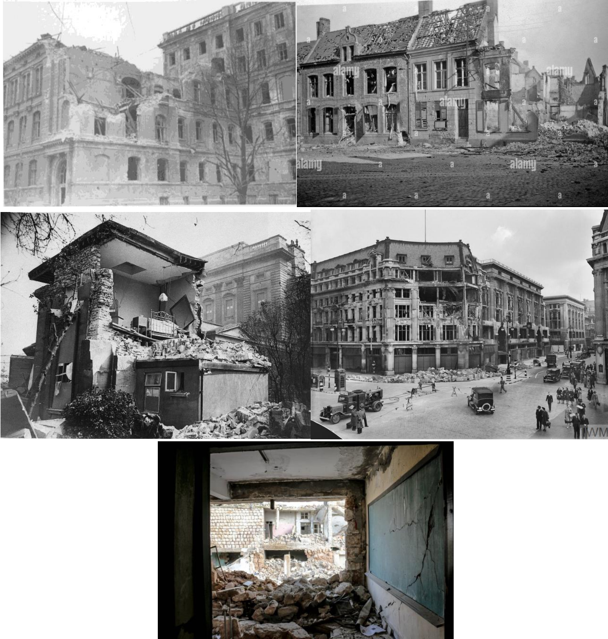
Figure 6: Contact Sheet for Destroyed Buildings and Streets [7, 8, 9, 10, 11]
